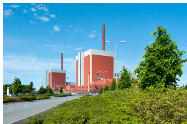
Figure 2. Olkiluoto nuclear power plant units 1 and 2. Source: TVO.
