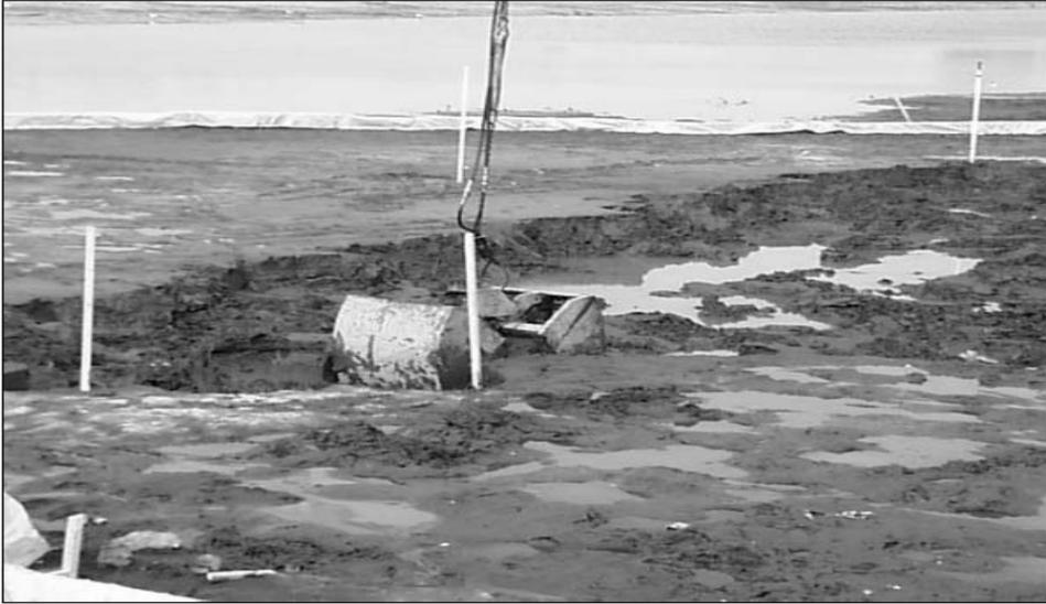
**Figure 5.** Excavation with a grab.
