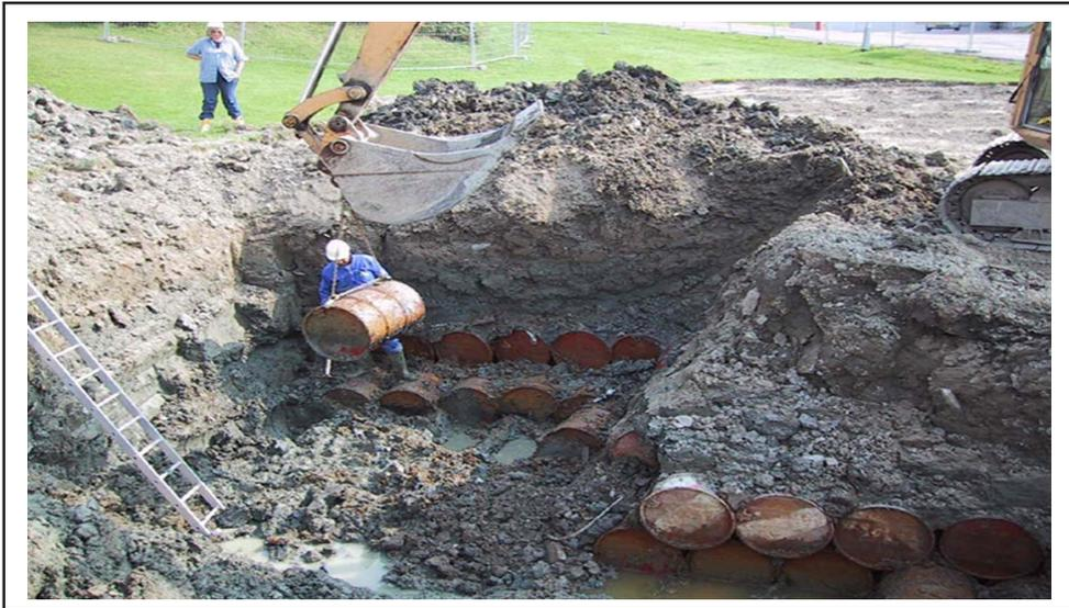
**Figure 1.** An excavator was used to lift the drums out of the repository.
