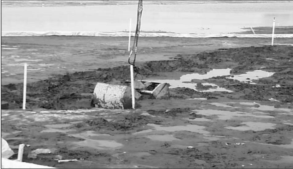
**Figure 5.** Excavation with a grab.
