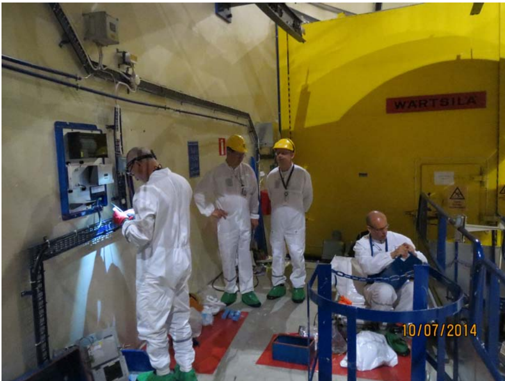
Figure 9. Installation of surveillance equipment for remote data transmission at the Loviisa NPP.
