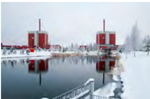
FIGURE 4. Olkiluoto nuclear power plant units 1 and 2. Source: TVO.
