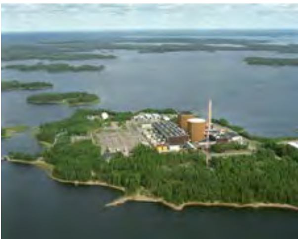
FIGURE 3. Loviisa nuclear power plant units 1 and 2. Source: Fortum.
