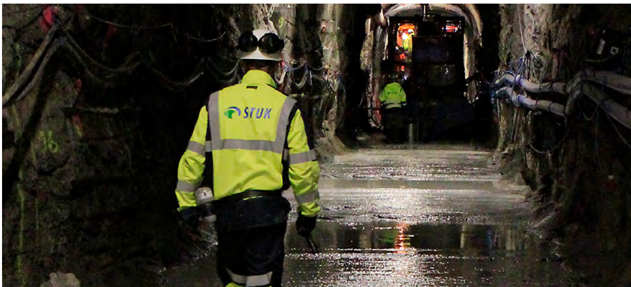
PICTURE 4: STUK oversees all phases of construction of the Onkalo at site. White liquide is drill cuttings waste generated during excavation of the bedrock. Picture: Paula Ruotsalainen/STUK.
