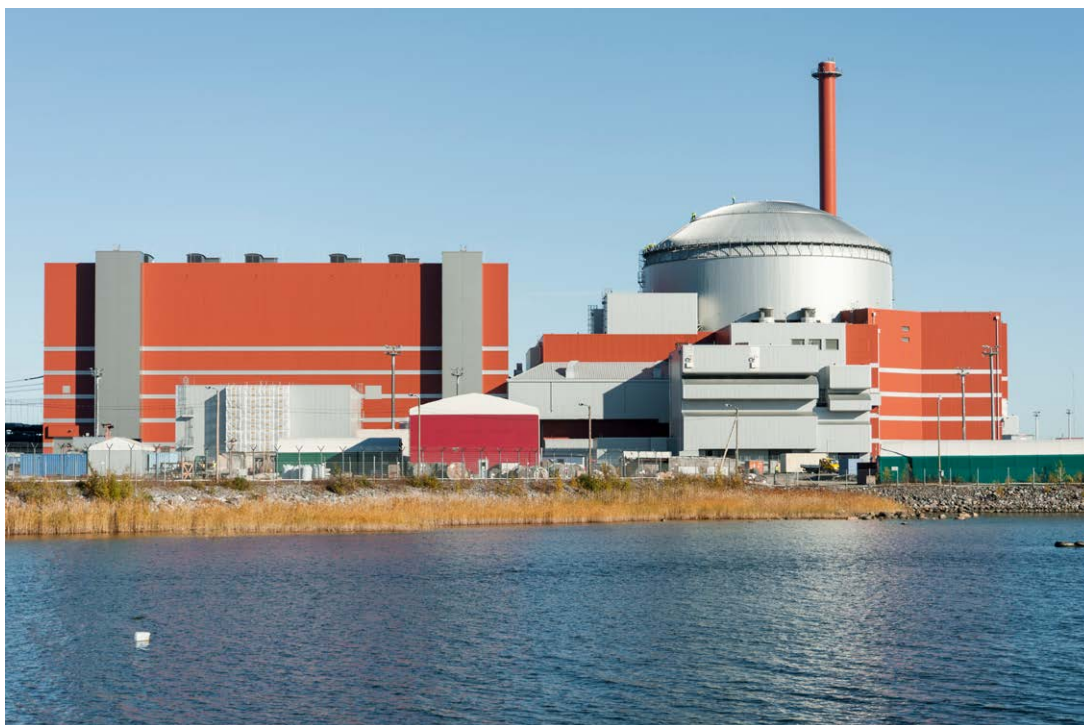
FIGURE 3. Olkiluoto NPP unit 3. Source: TVO.
