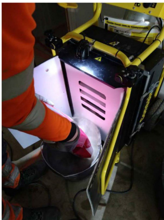
Figure 1. Use of a directed air cleaner in the mixing of mortar.
